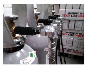
Step 2 Connect the 4 female ends of the 3/8 hoses to the male connectors on the distribution block.
